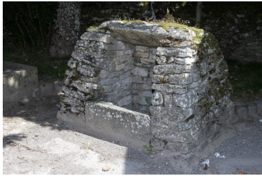
Puits. Phot. Denis Pillet IVR52_20084401852NUCA
