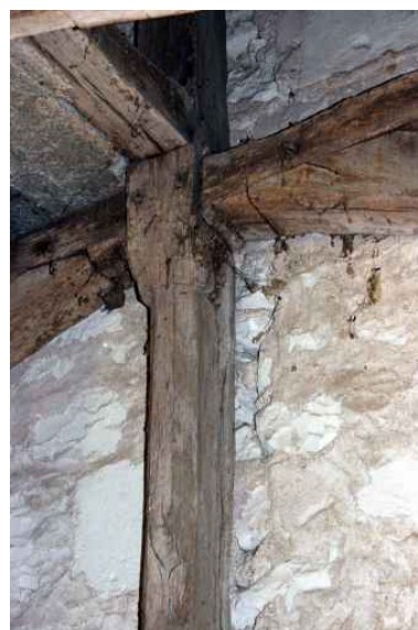
Le logis, charpente : assemblage. Phot. Jean-Baptiste Darrasse IVR52_20067205953NUCA
