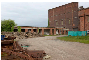
Extension de 1930. Phot. Denis Pillet IVR52_20134401483NUCA
