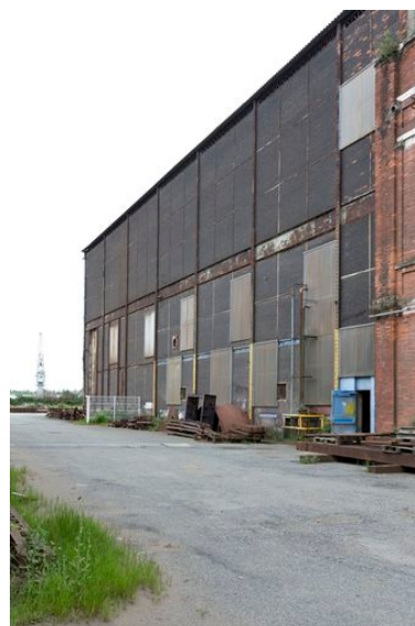
Chaufferie. Phot. Denis Pillet IVR52_20134401461NUCA
