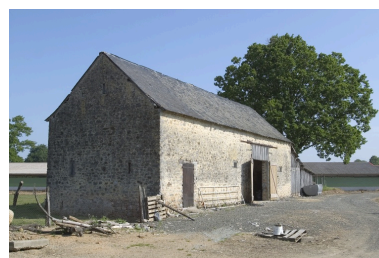
L'étable (?). Phot. François Lasa IVR52_20045301839NUCA
