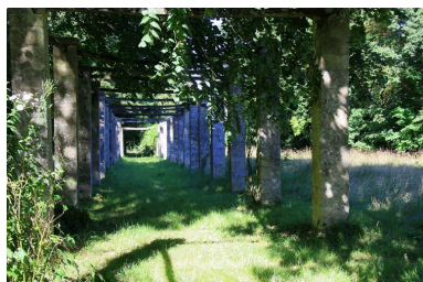
La pergola. Phot. Jean-Baptiste Darrasse IVR52_20087201493NUCA
