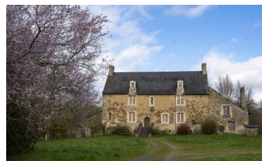
Le logis. Phot. Pierre-Bernard Fourny IVR52_20225300329NUCA
