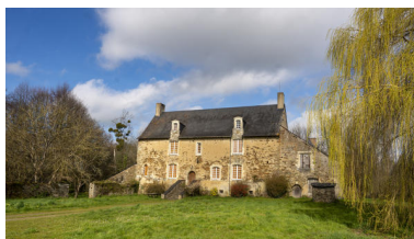
Le logis. Phot. Pierre-Bernard Fourny IVR52_20225300302NUCA
