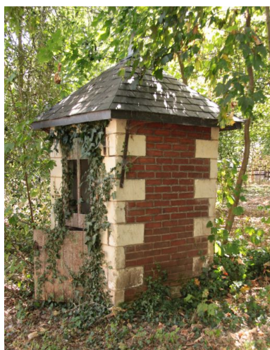
Latrines. Phot. Jean-Baptiste Darrasse IVR52_20097200500NUCA
