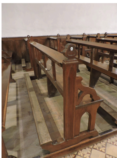
Bancs de la nef. Phot. Yannis Suire IVR52_20218501737NUCA
