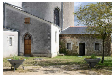
Communs. Phot. Armelle Maugin IVR52_20254900633NUCA
