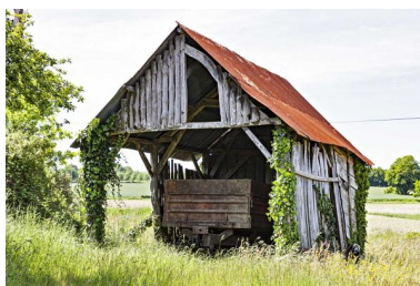
Loge-remise du Boulay. Phot. Yves Guillotin IVR52_20215300677NUCA
