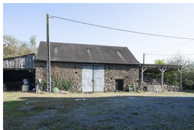
Remise (2023 ZC 132). Phot. Yves Guillotin IVR52_20185300427NUCA
