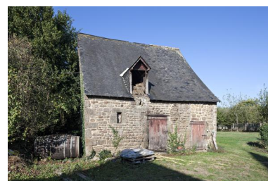
Etable-fenil (2023 ZC 132). Phot. Yves Guillotin IVR52_20185300426NUCA
