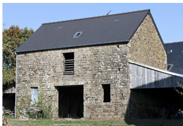
Etable-fenil (2023 ZC 104). Phot. Yves Guillotin IVR52_20185300443NUCA
