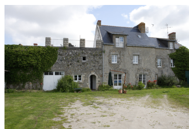
Logis. Façade sud. Phot. Denis Pillet IVR52_20084401612NUCA
