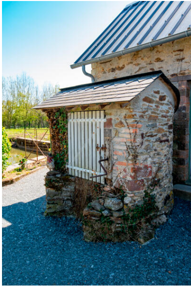
Le puits. Phot. Pierre-Bernard Fourny IVR52_20235300327NUCA
