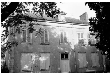
Elévation principale. Phot. Marie-Anne Eon IVR52_19724900384Z
