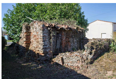
Four debout Huteau, village des Tuileries. Phot. Denis Pillet IVR52_20154400404NUCA
