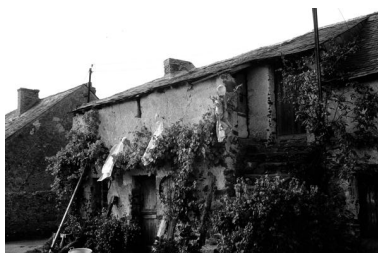
Elévation principale, 1972. Phot. Marie-Anne Eon IVR52_19724900417Z
