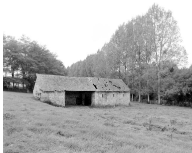
La remise. Phot. François Lasa IVR52_20015300551X
