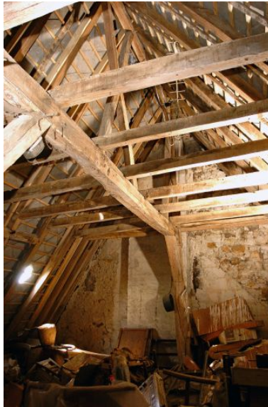
Charpente. Phot. David Huard IVR52_20047205456NUCA
